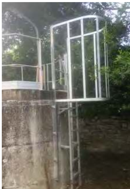
Crinoline barre antichute STEP route de Corzé
